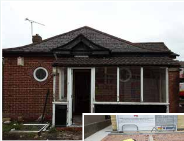
Before work commenced
