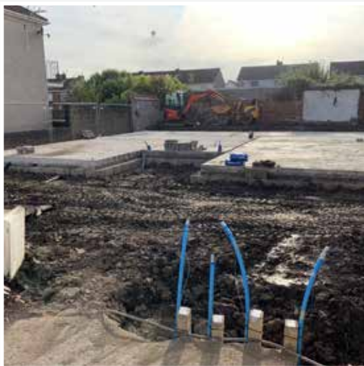
Foundations are in place
