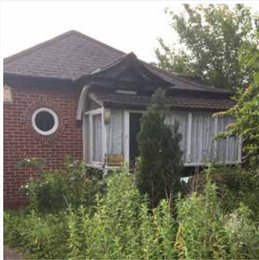
Before work commenced
